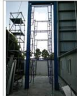
Frame scaffolding assembly
